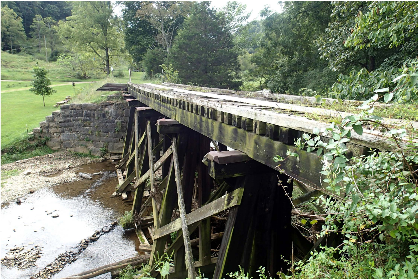
Railroad trestle over Abrams Creek, ©Rick Heppert
